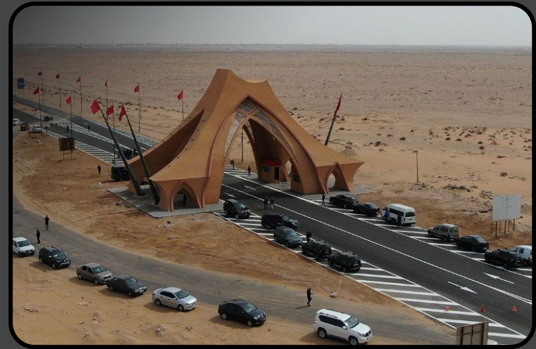
Tiznit-Dakhla Expressway (Right)
